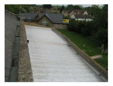
The new church roof, finally finished. At the moment it is shiny stainless steel but is expected to weather to a dull lead coloured appearance.
